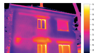
Thermal image with ScaleAssist
